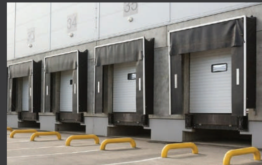
LOADING HOUSES & DOCK LEVELLER
